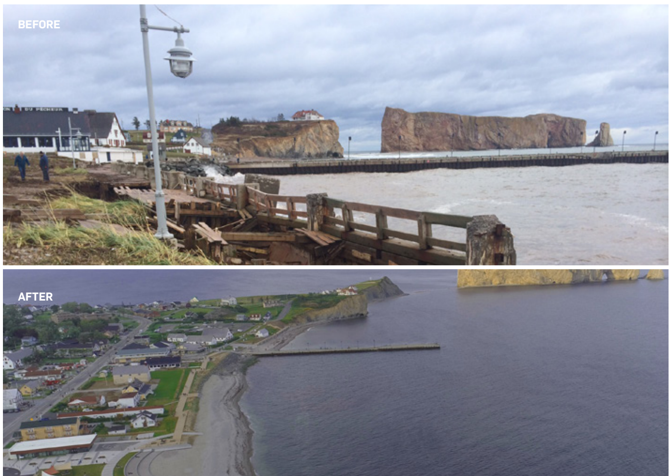
Image 4. Before and after the beach replenishment to protect Percé coast in Québec (Credit: Ville de Percé)
