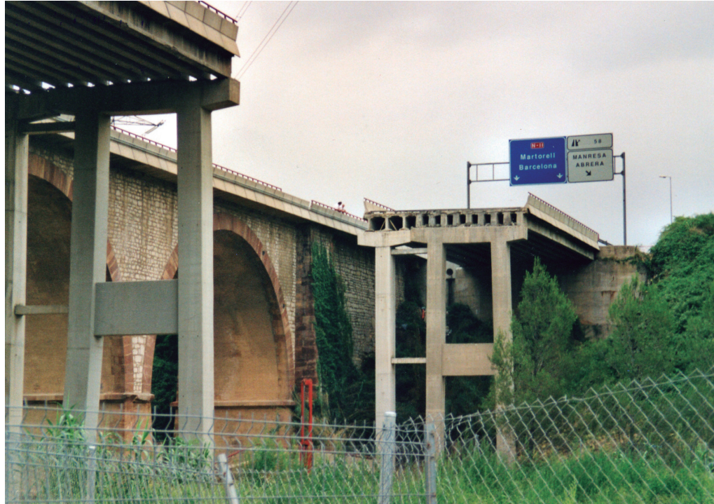
A bridge on the N-II highway destroyed after the flooding of 10 June 2000.
